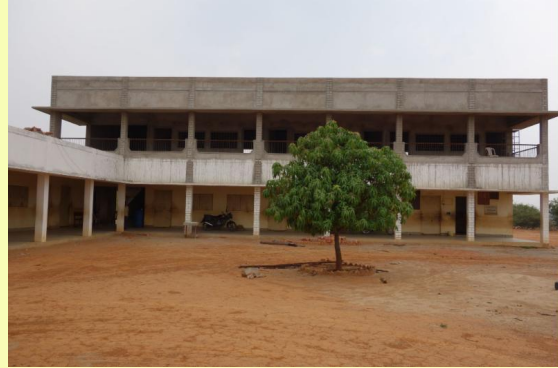
Turkahan school today with a new middle school extension being built
